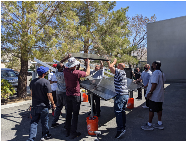
SECTOR participants with Paving the Way in Lancaster complete their final day of a 40-hour training in solar panel installation with Glenn Bland Solar.
